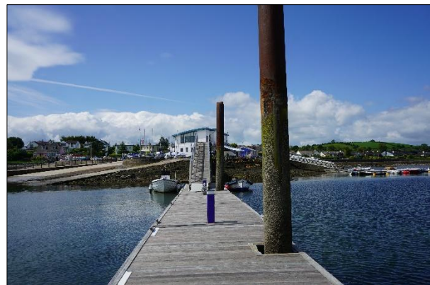
Plate 1.2: The Site – the floating pontoon & guide piles at low water; SLYC on-shore compound to the rear of frame [June 2025]
