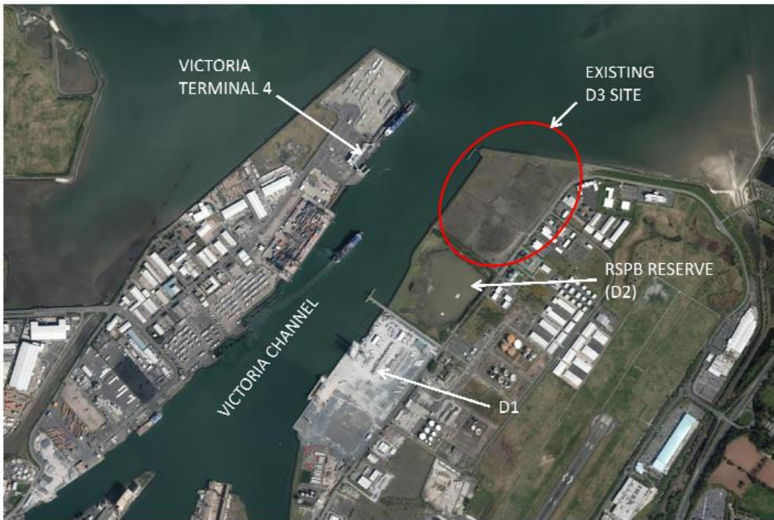
Aerial view of the D3 site
