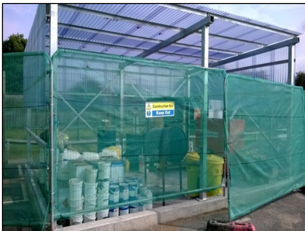
Figure 4: Examples of bunded and covered COSHH areas and containers
