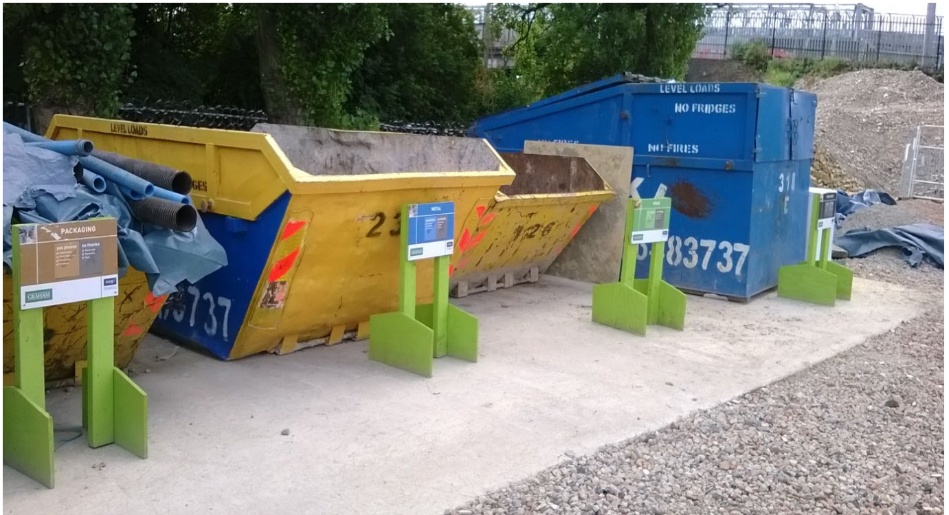
Figure 15: Waste Storage Arrangements
