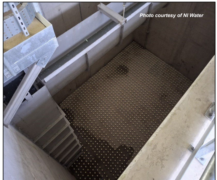
Figure 2 - 8 Ballinrees WTW GAC Filter Construction
