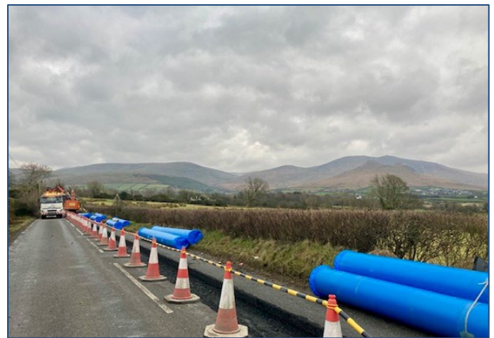
Figure 2 - 7 New Mains Installation
