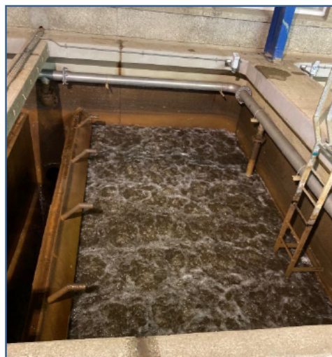
Figure 2 - 2 Backwashing a Filter
