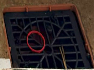
Image: Drinking Water Quality Sampling Point at a Service Reservoir
