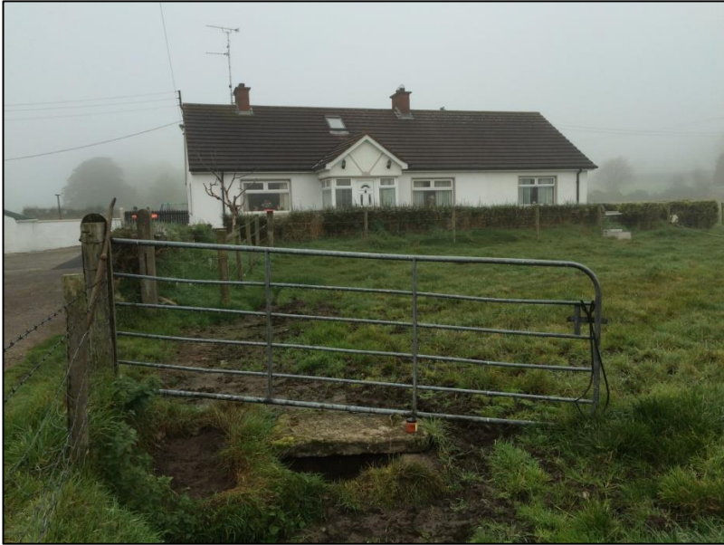
Dye test done at ST of 22 Mulnafye Road 02/10/15
