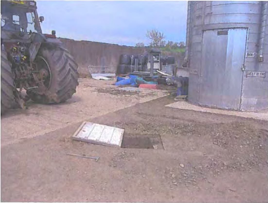
Inspection chamber adjacent to slurry tank.
