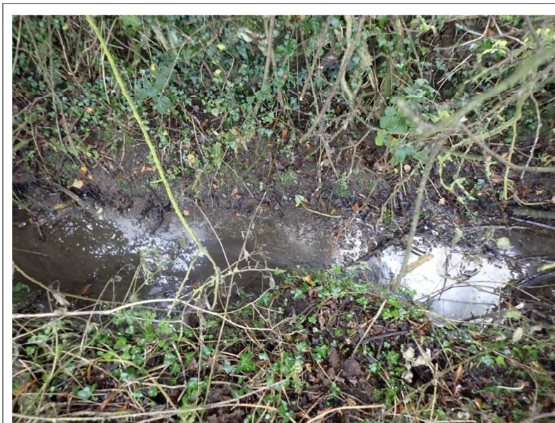
Photo 16. Drainage channel along Hedgerow H4.
