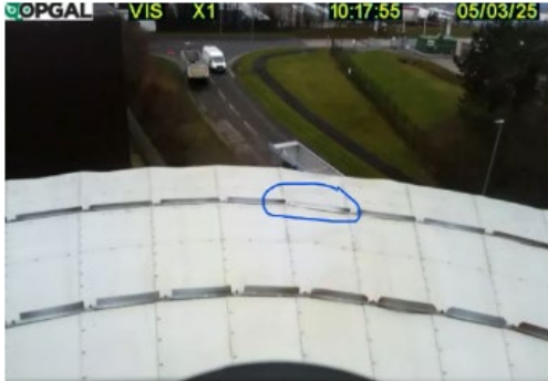
Top of Digester 1 roof emission location
