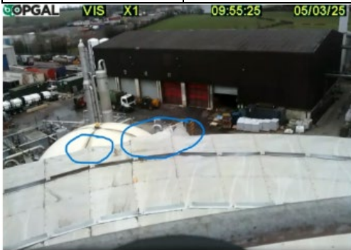
Top of Digester 2 roof emission locations
