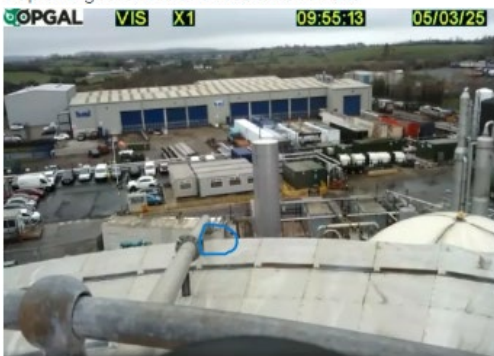
Top of Digester 2 roof emission location
