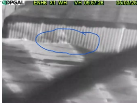
Top of Digester 2 back of roof emission location
