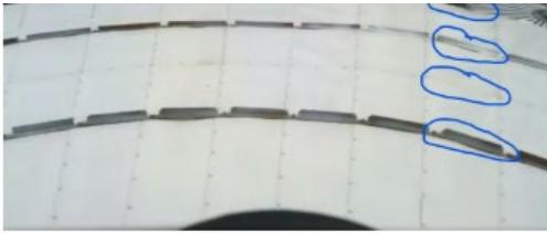
Top of Digester 1 roof - emission locations
