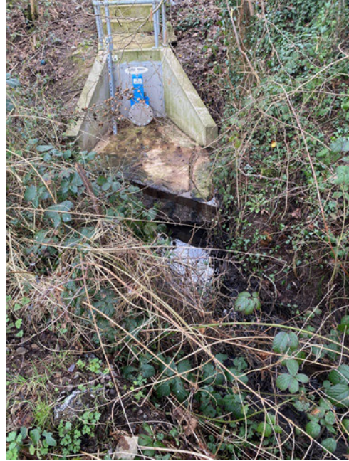
Photo 8 Surface water discharge point
