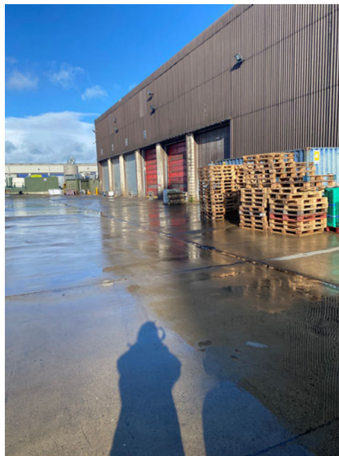
Photo 3 Doors all closed on intake bays
