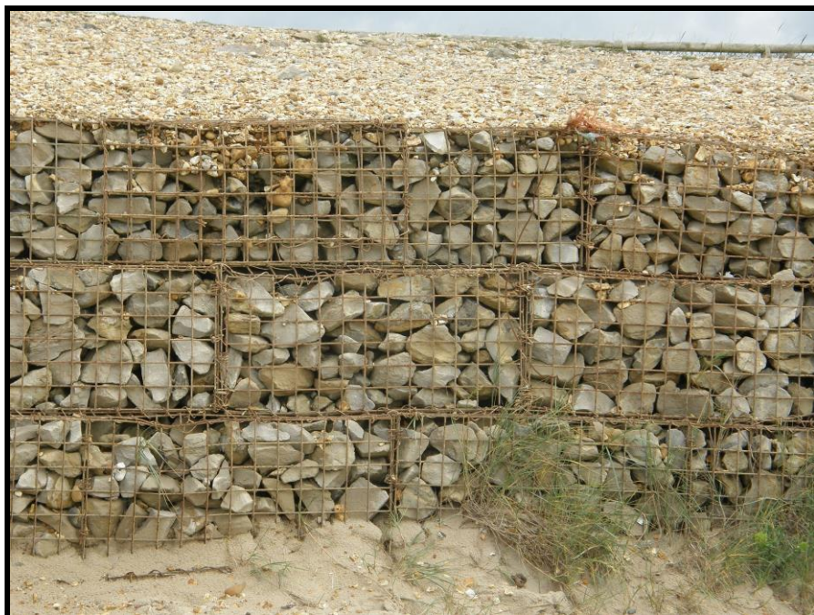
Figure 28 Large-scale Rock gabions for coastal defence (source: https://commons.wikimedia.org/wiki/File:Gabion-hengistbury-head.JPG )
