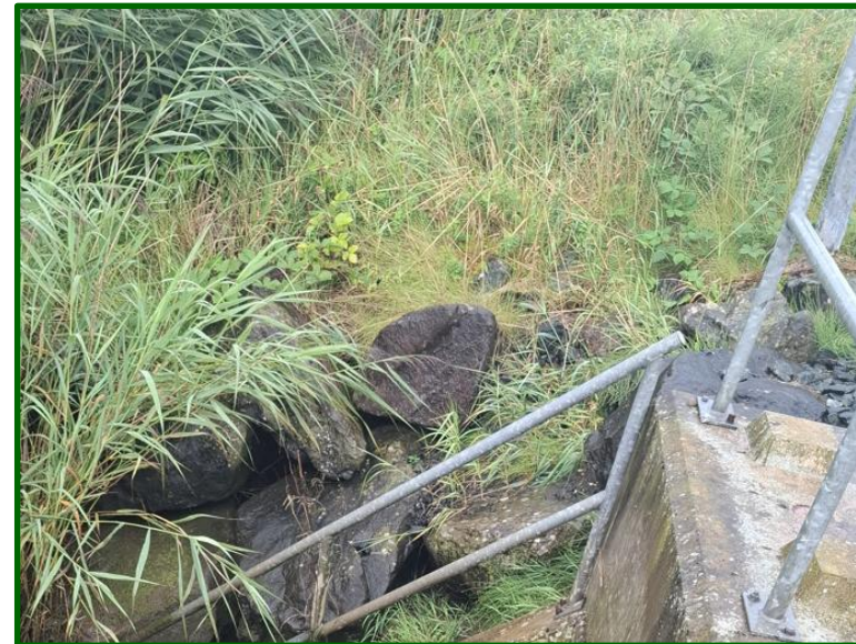
Picture 8: Existing Sea Defences covered, with minimal amounts of vegetation (J3.5)
