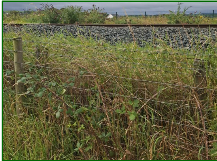
Picture 9: Fence (J2.4) noted running along the northern boundary of the site compound
