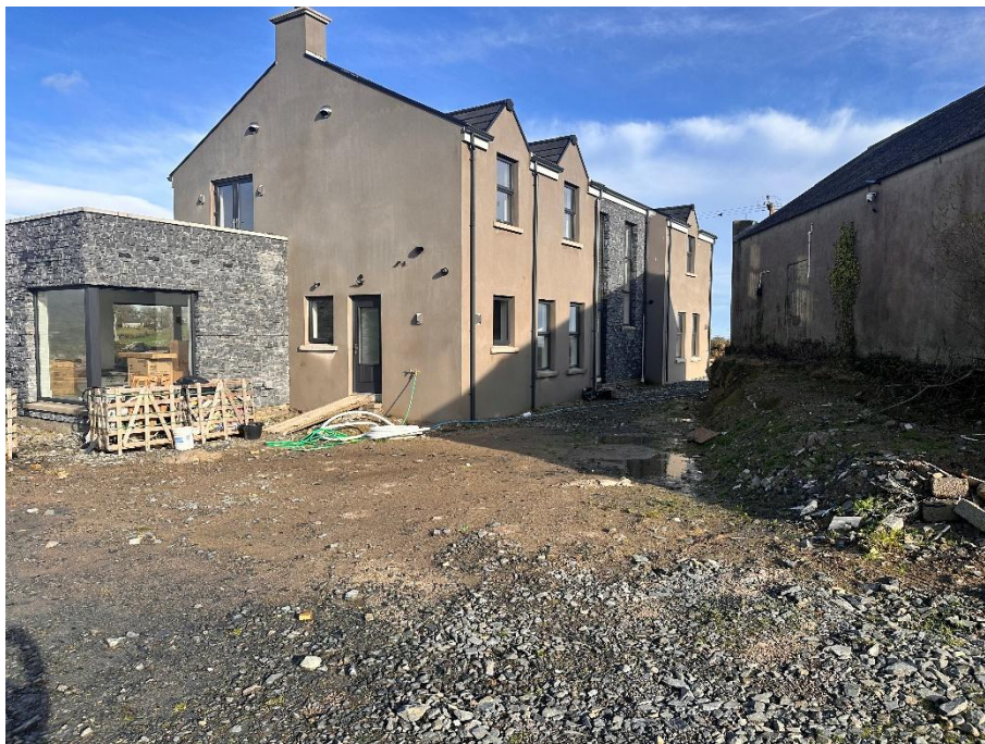
Photograph 4: Newly constructed dwelling
