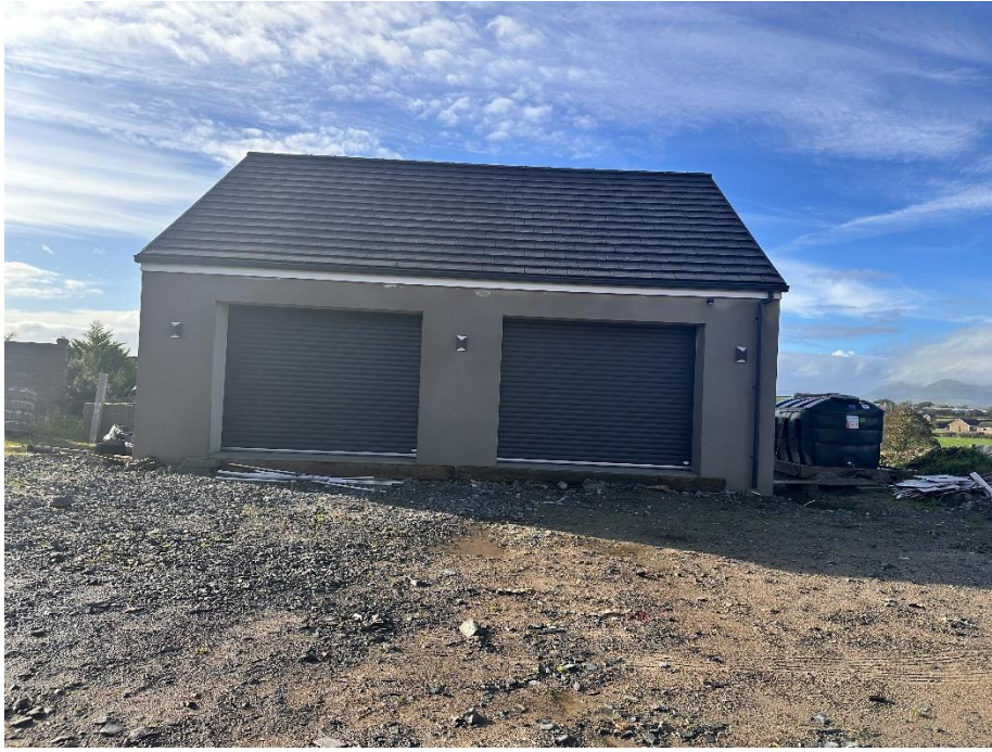
Photograph 5: Newly constructed garage
