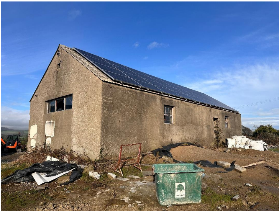
Photograph 6: Outbuilding 1 to the south of the dwelling
