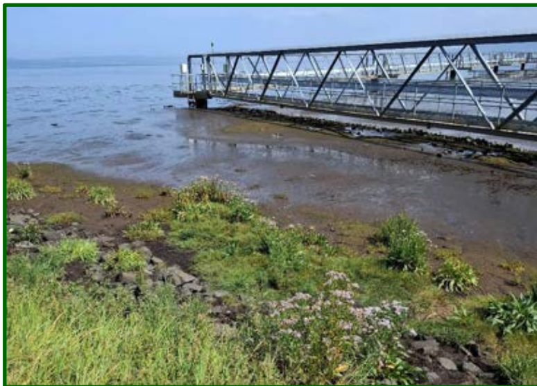
Picture 7: Buildings/Structure (J3.6) – metal walkway on-site
