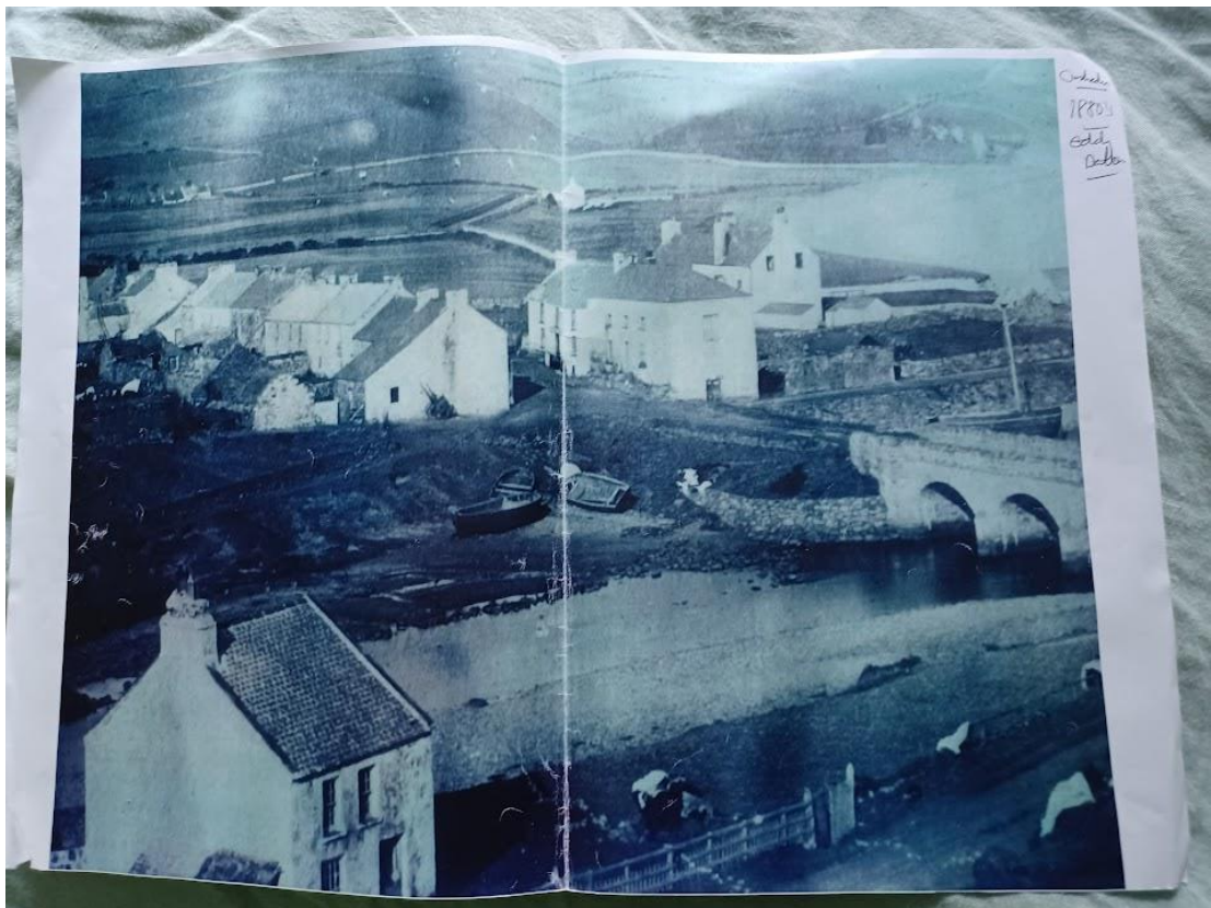
Photograph A3.2 Upstream side of Cushendun Bridge late 1880s (from Kirk McClure Morton, 1988)
