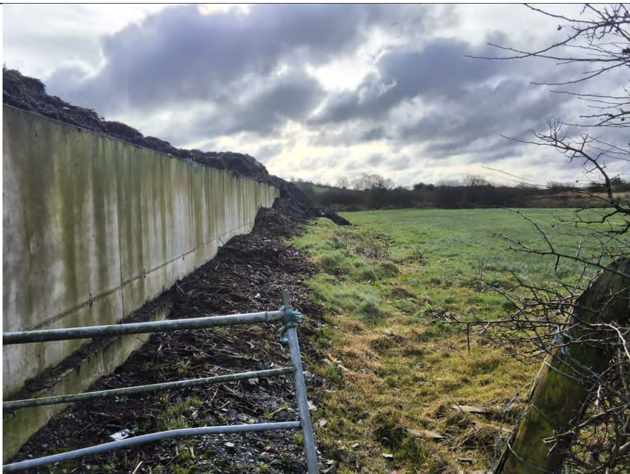
Figure 8 Site material being deposited outside the sites boundary.
