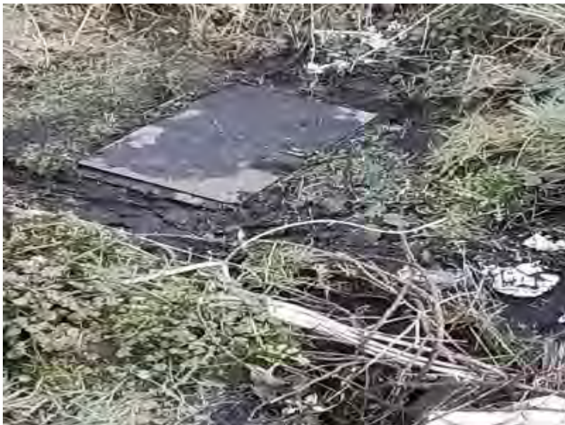
Figure 6 Access hatch to culverted stream on sites NNE boundary.
