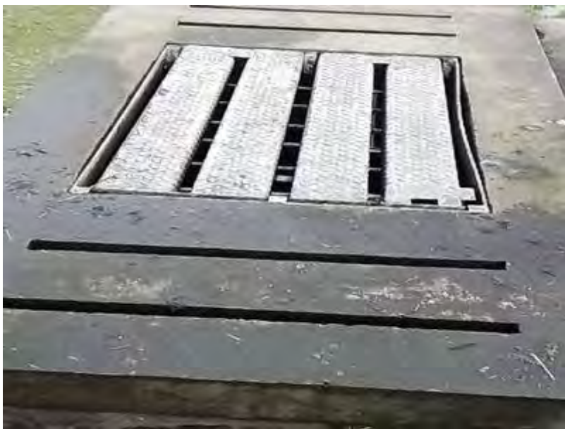
Figure 2 Access hatch to culverted stream. Eastern boundary of site.
