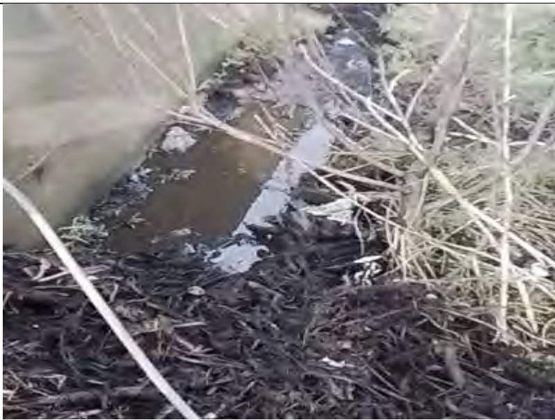
Figure 3 Signs of previous untreated dirty water escaping from site confines.
