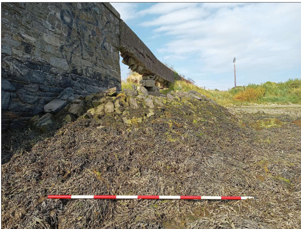
Figure 11: Photograph of the battered stone buttress/foundation to the base of the embankment/causeway below the parapets and abutment facing northeast
