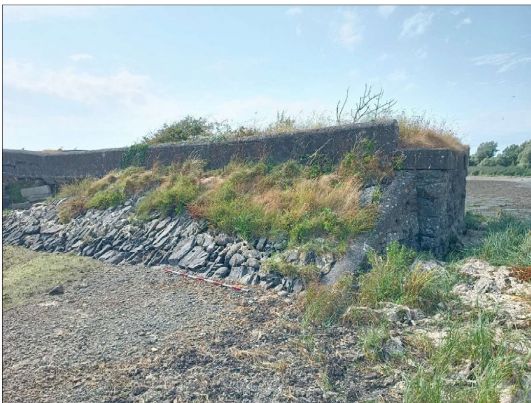
Figure 13: View of section of supported parapet and northeast abutment, facing northeast
