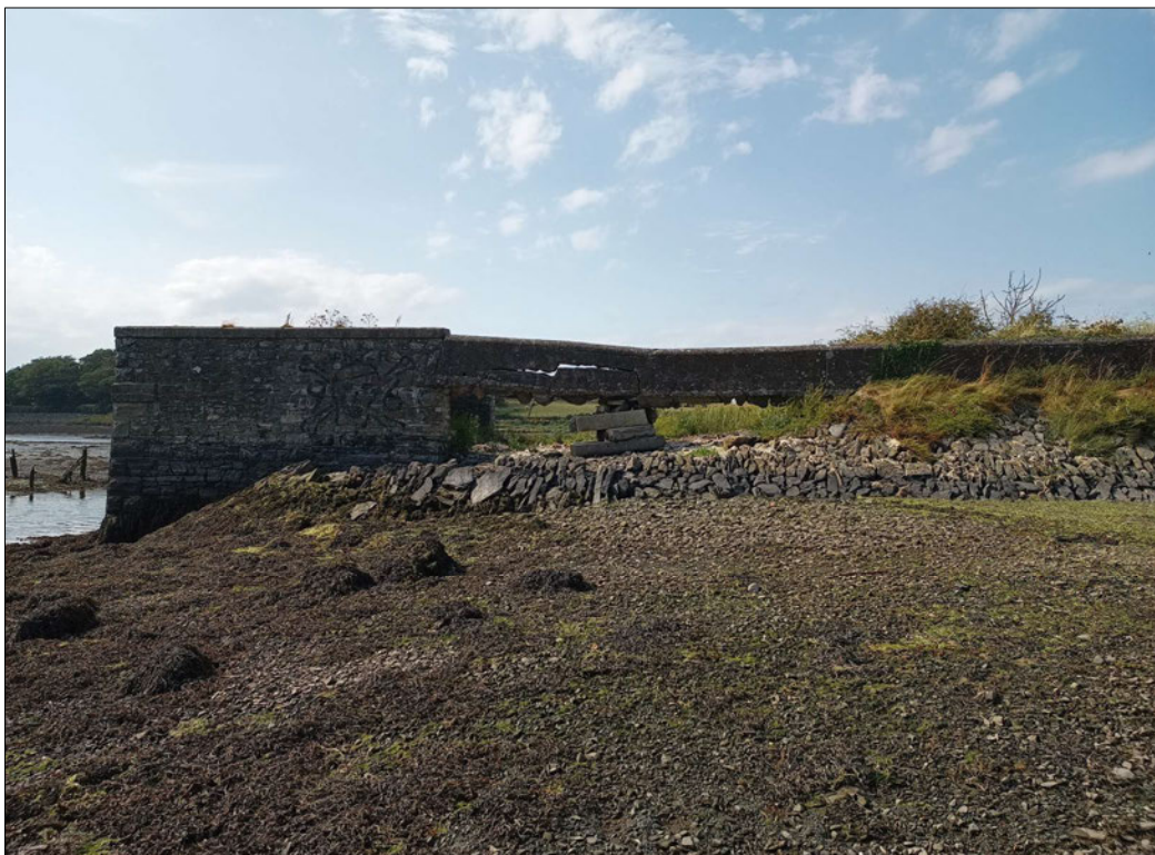
Figure 10: Photograph of the stone embankment/causeway below with the parapets suspended between the stone abutments, facing northwest
