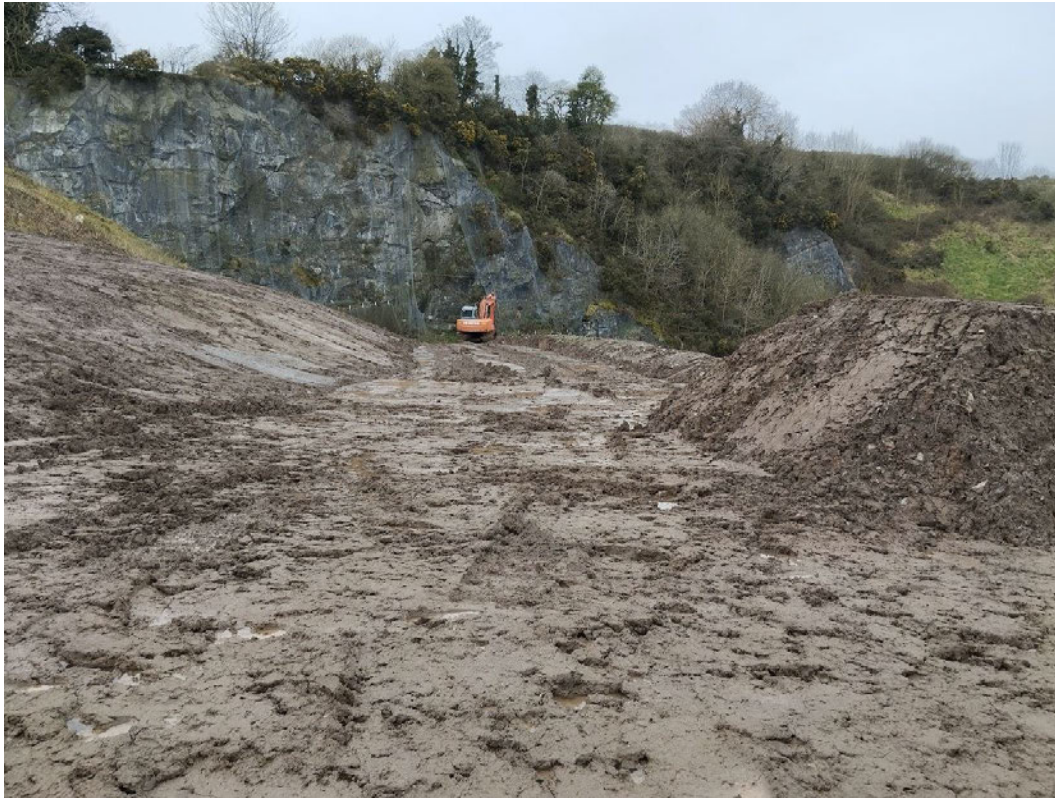
Figure 1.1 – Compacted Clay Bund
