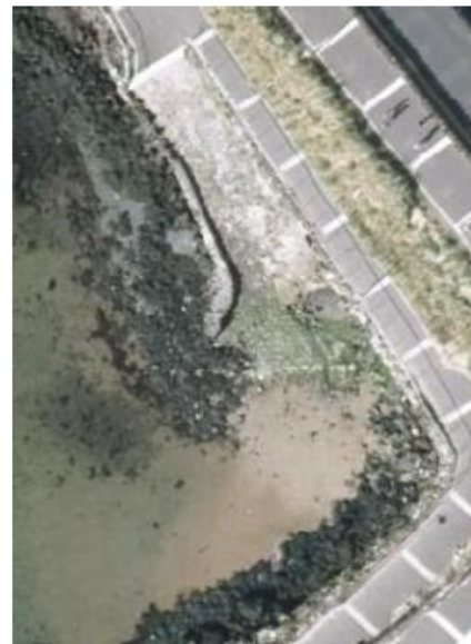
Figure 2.2: Old Slipway Aerial Photograph (from OSNI)
