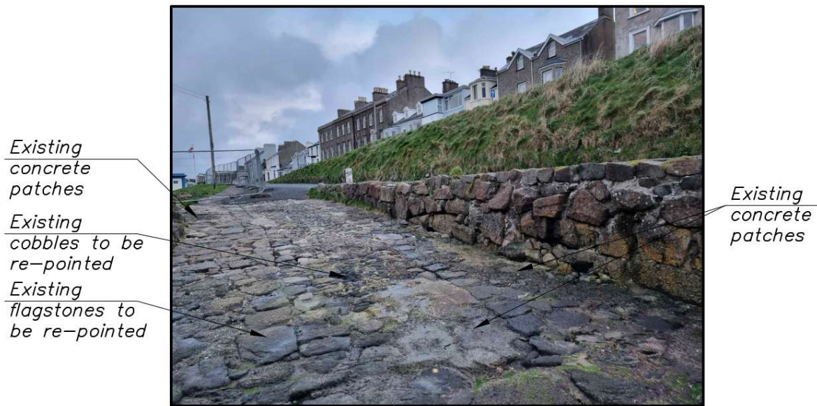
Figure 1. Existing Slipway Surface
