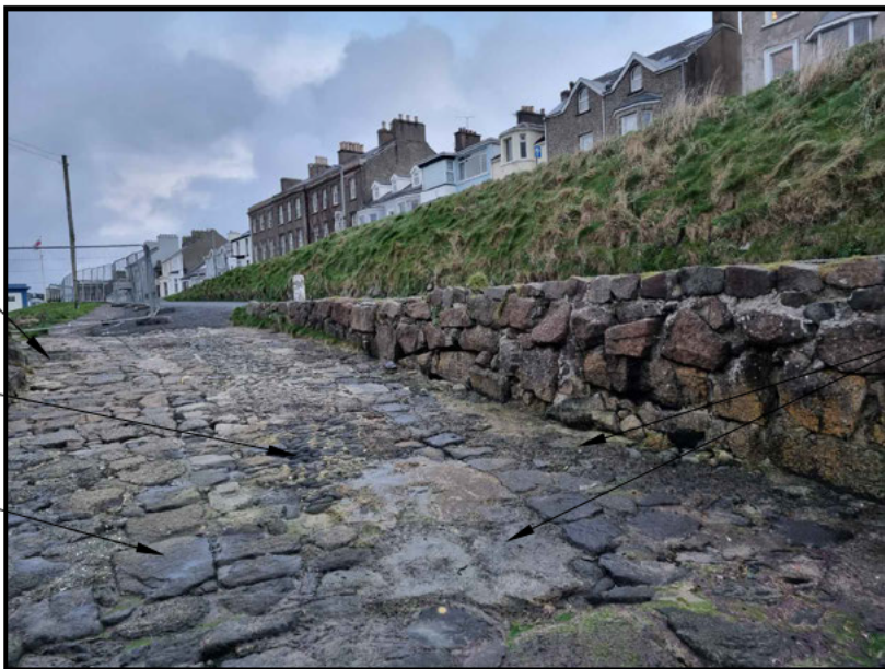
Existing concrete patches
