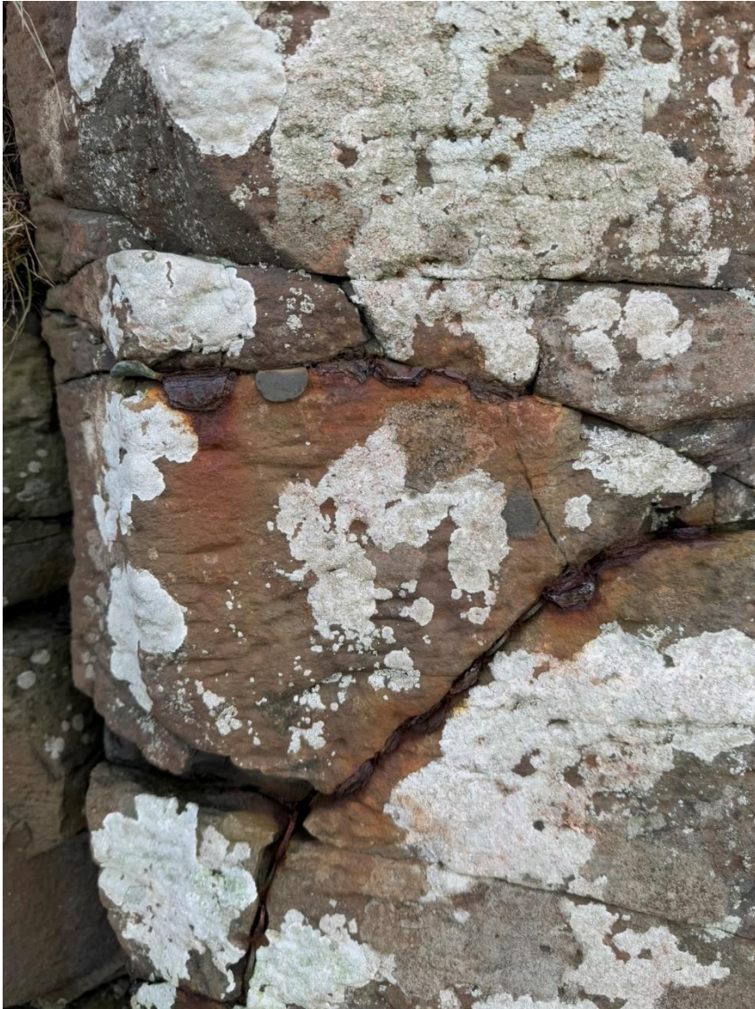
Figure 5. Coins hammered in to joints
