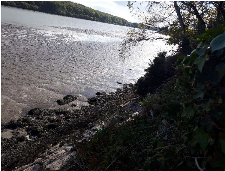
Figure 4 – Mudflats – temporary working platform to be placed on top of mudflats with geogrid separator layer
