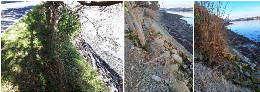
Figure 3 – Existing rock armour section
