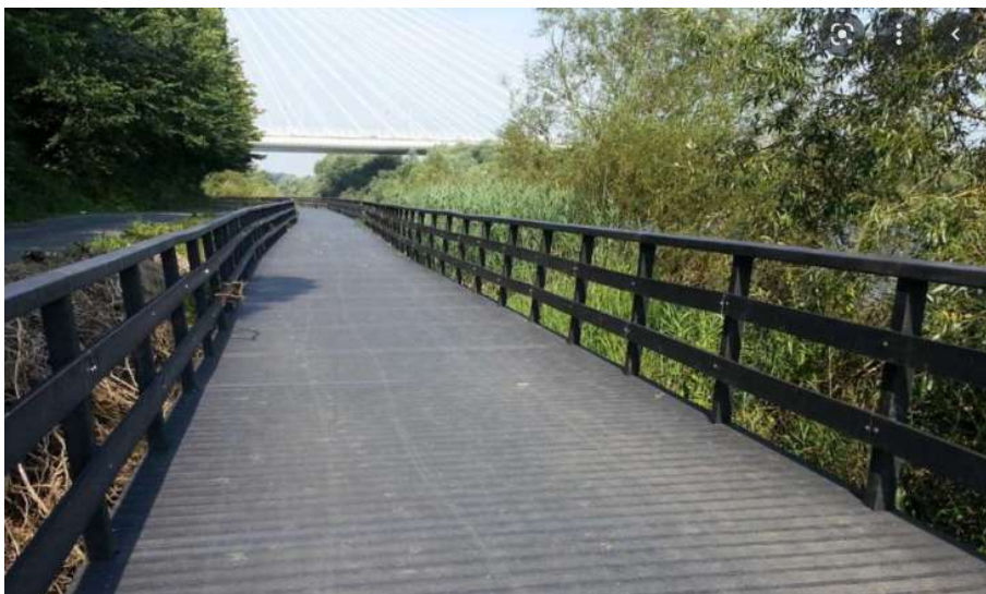
Figure 6 – Example of piled boardwalk
