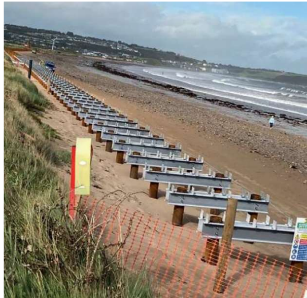
Figure 5 – Example of piled boardwalk
