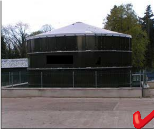
Well maintained above ground slurry tank
