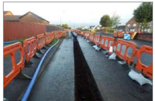
Figure 2.8: New Mains Installation
