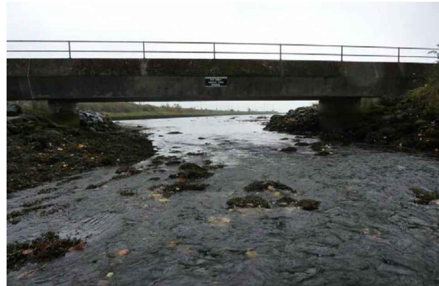
Photo 1 - View of the structure from upstream
