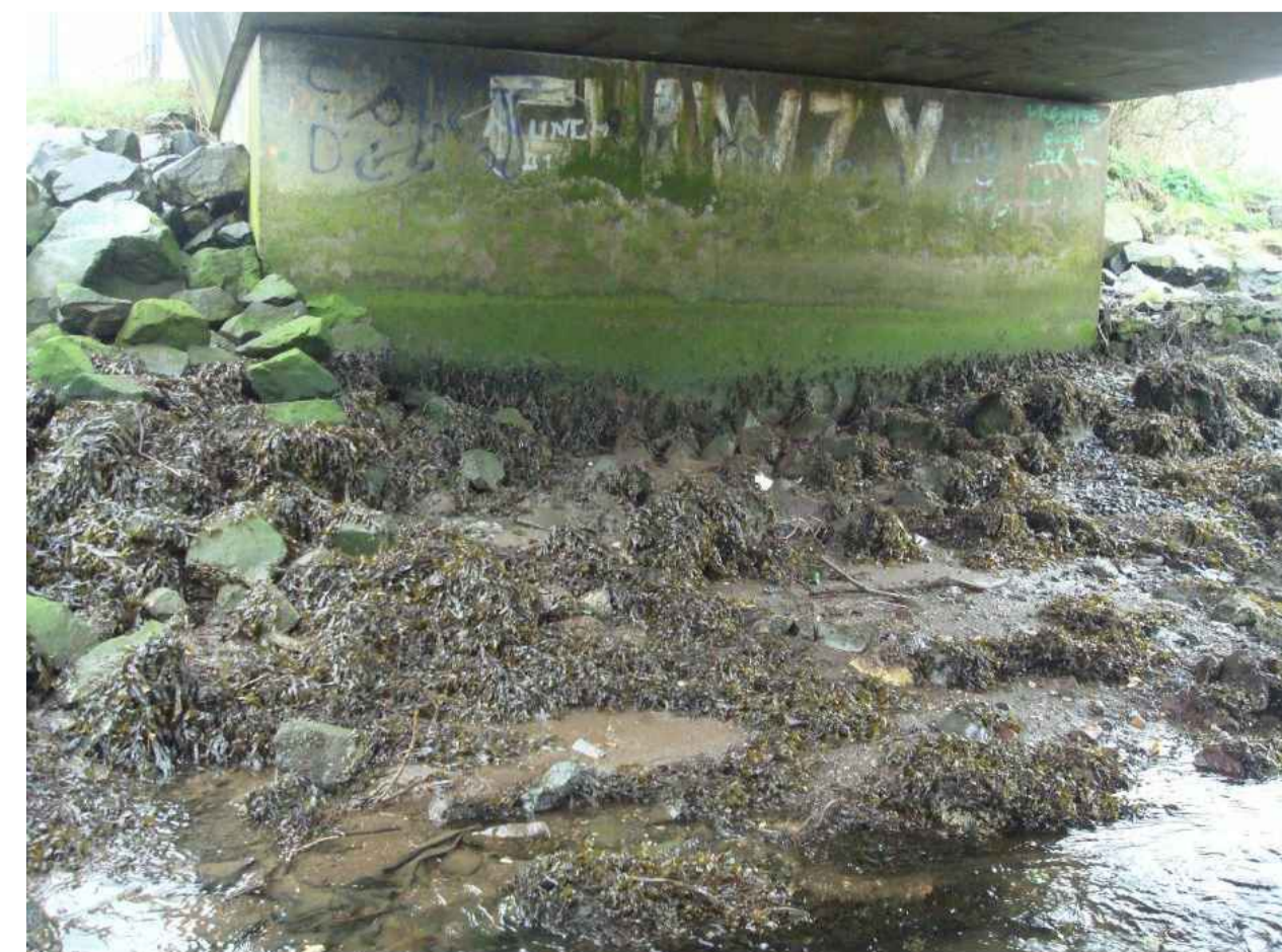
Photo 3 - Loss of rock armour at High Mileage abutment
