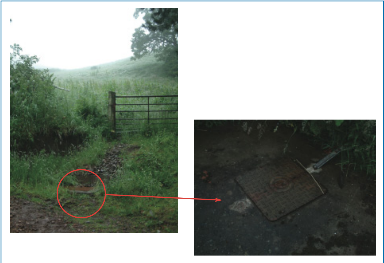
Figure 5.15 Chamber where pipework from sources A1 and A2 are considered to join
