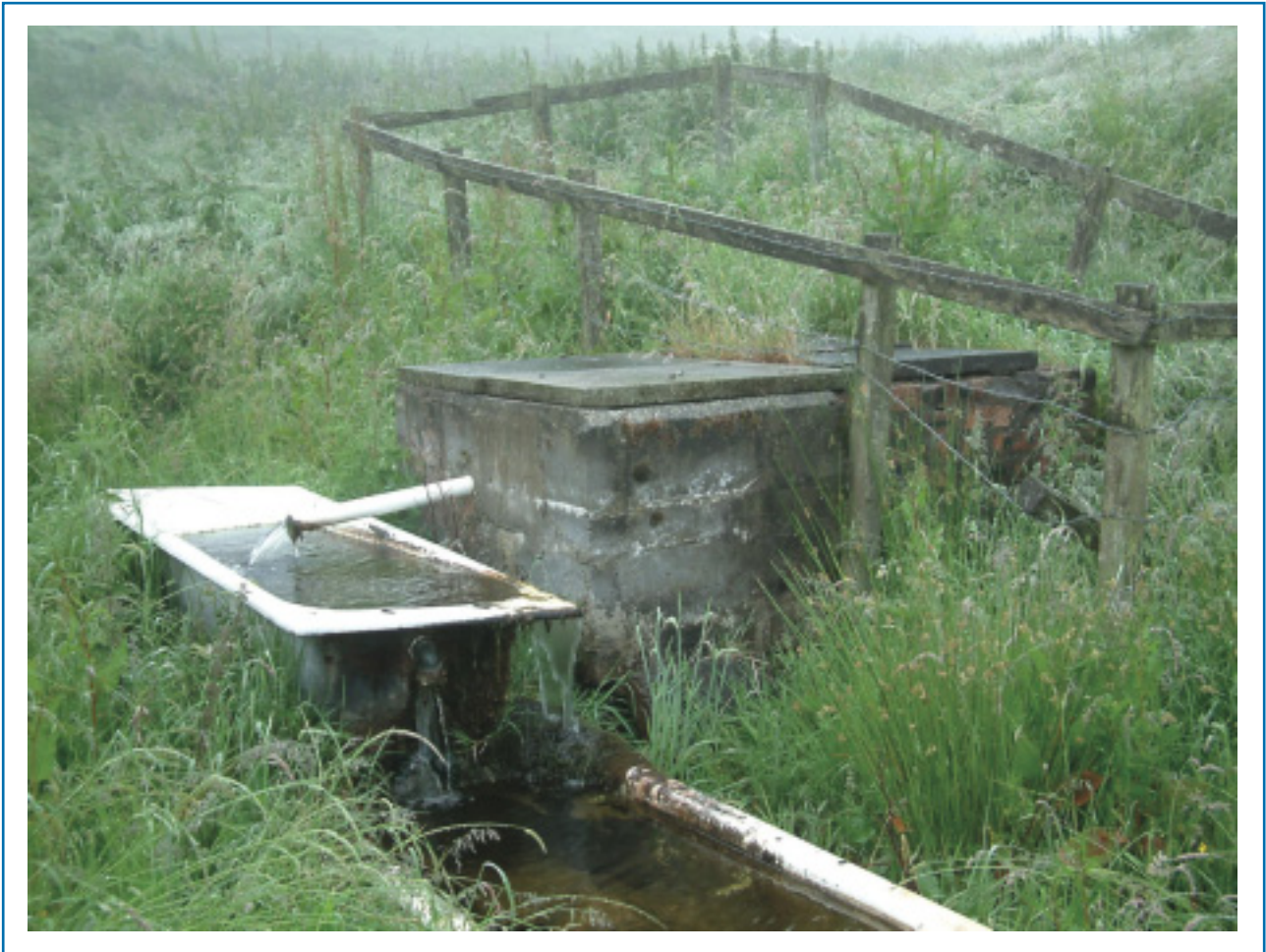
Figure 5.8 General situation encountered at source A1 (Weathertop)
