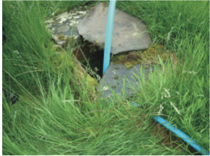
A7 – intermediate collection/storage tank
