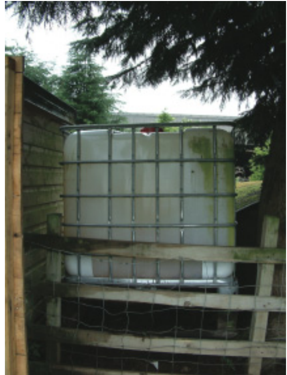
Chlorine reserve at Tank B1
