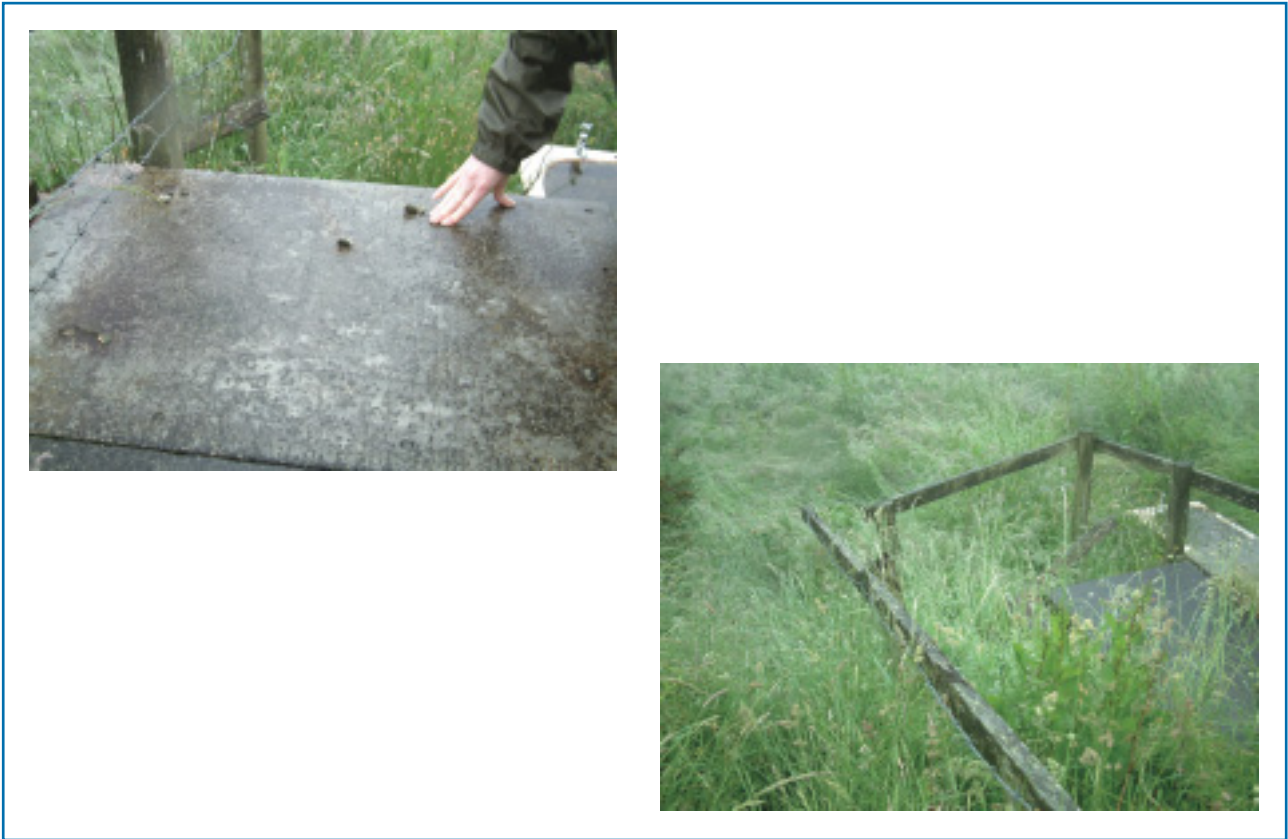
Figure 5.9 Evidence of faecal material deposited on top of collection tank at site A1
