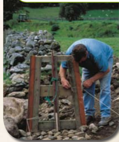
Building a dry stone wall
