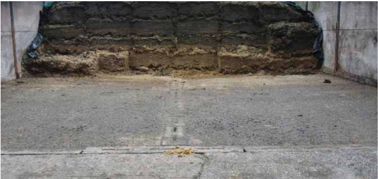
Photo 8: Run-off from a well managed silo with minimal silage droppings and no effluent present, could produce dirty water. Where effluent is present slurry is produced.
