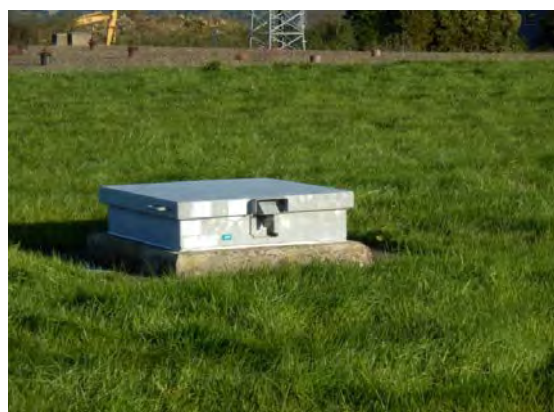
Figure 4.2: Protective cover on access point to Service Reservoir
