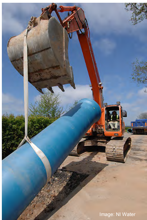
Figure 4.5: New Mains Installation
