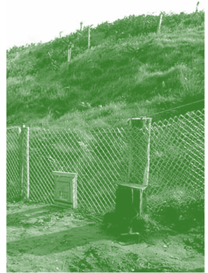
Exclusion Fence & Badger Gates
