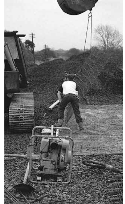
Reinforcing roof of Sett
