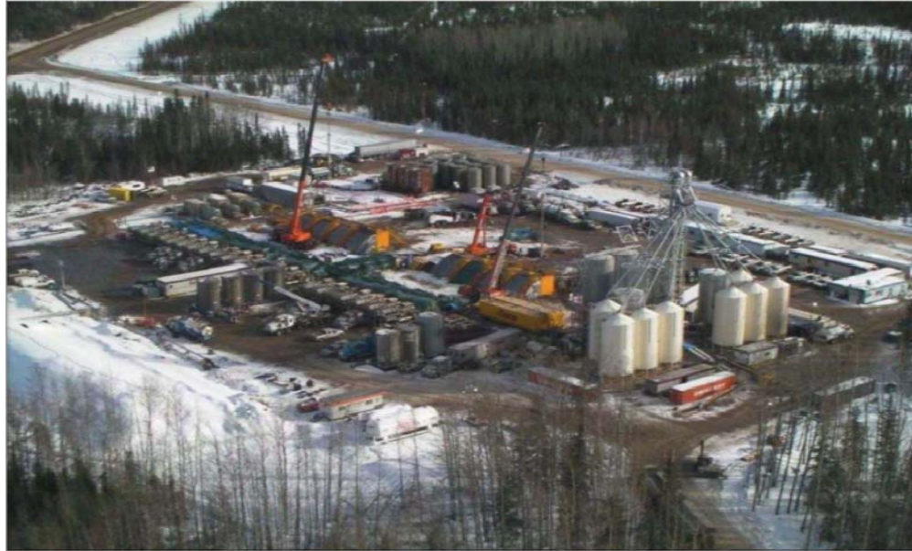
“Super-fracking” pad – 24 wells per pad – one every 2 miles
