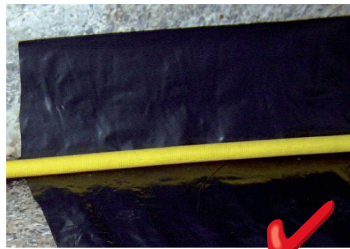
Photo 9 – Protecting silage pit wall-floor joints
