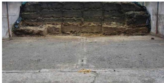
Photo 31 - Run-off from a well managed silo with minimal silage droppings and no effluent present, could produce dirty water. Otherwise, where effluent is present, it should be managed in the same way as slurry.
