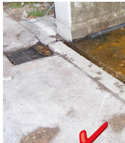
Photo 13 – Silage clamp with well maintained channels draining to effluent tank
