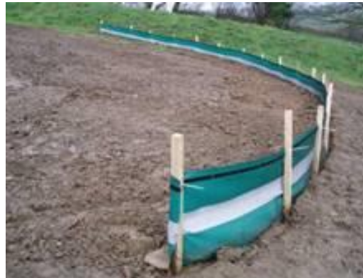
Photo 20 – Sediment fencing
