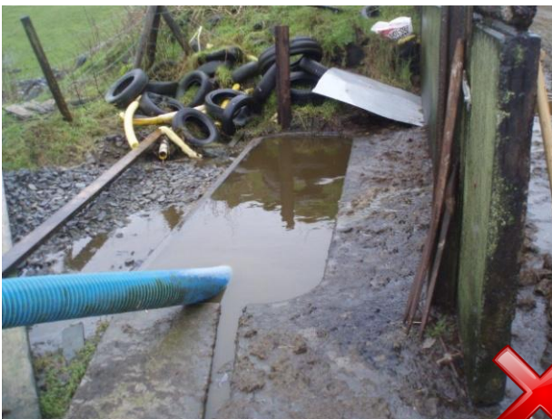
Photo 12 – Overflowing effluent tank not being managed
