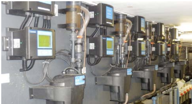
Figure 3.4: On-line Turbidity Monitors
