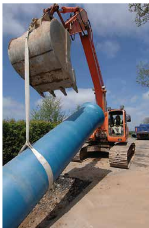
Figure 4.5: New Mains Installation
