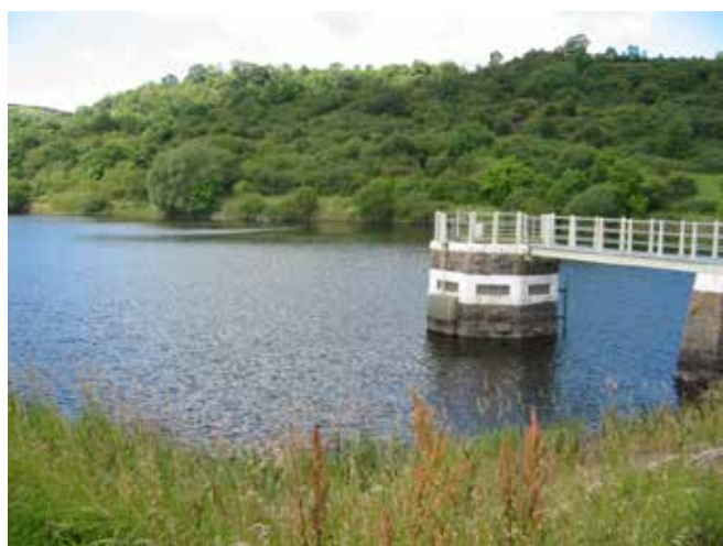
Figure 2.1 Raw Water Abstraction Point
